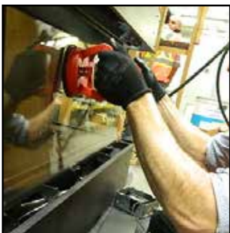
Handle glass with supplied vacuum clamps
