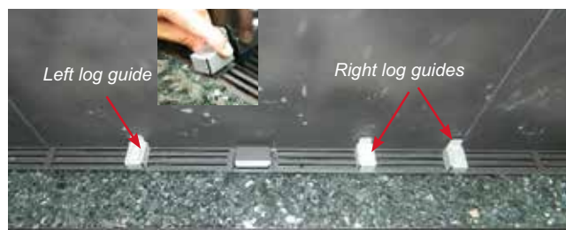
Log guides installed
