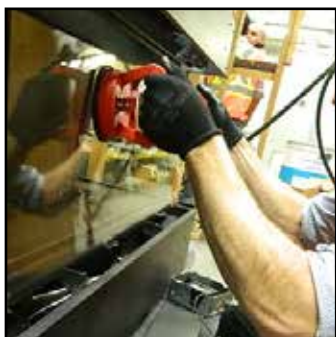
Handle glass with supplied vacuum clamps
