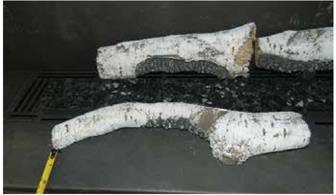
Log 4 —2" to end of front panel
