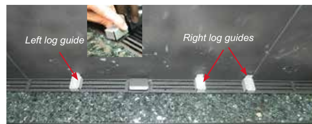
Log guides installed
